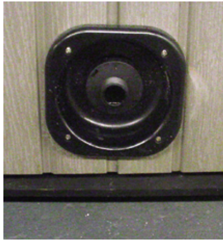
Figure 18. Cabinet mounted drain valve
