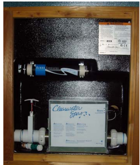
Figure 1-2 – Controller, Ozonator and Drain Valve
